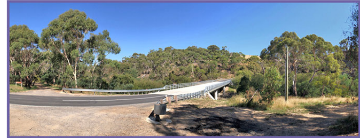
Slate Quarry Road Bridge
