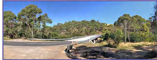
Slate Quarry Road Bridge
