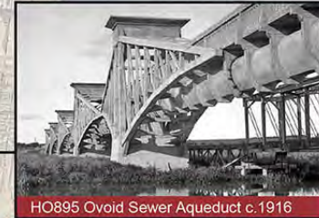
HO895 Ovoid Sewer Aqueduct c.1916
