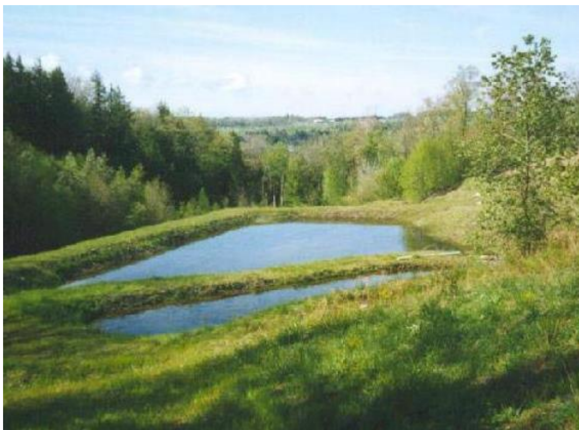
Figure B-9 Vertical flow wetland
