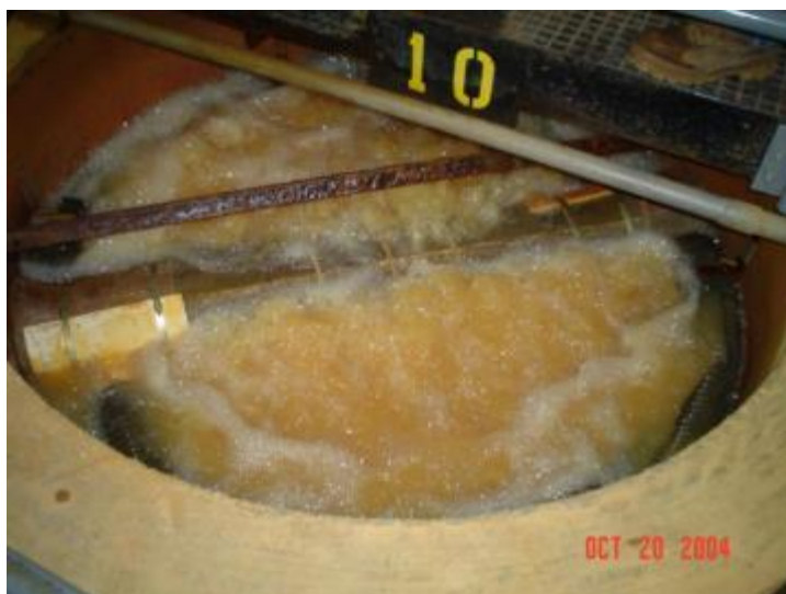
Figure B-2 Limestone diversion well
