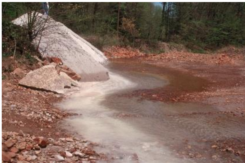
Figure B-1 Limestone sand placed along a polluted stream
