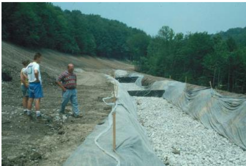
Figure B-4 ALD under construction
