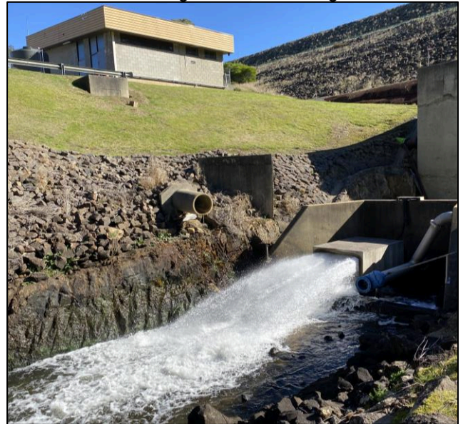
Figure 3. Environmental water (9ML/day) being released from Lal Lal Reservoir on May 12 2021 (Photo: R.Glover)
