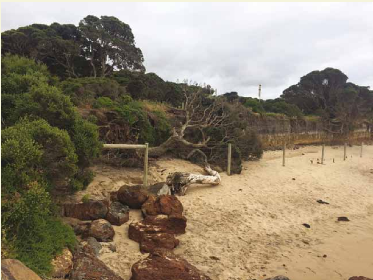
Erosion along Point Roadknight beach, Anglesea.
