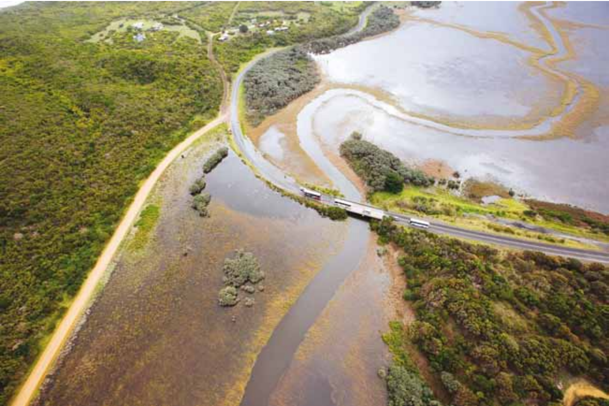
Flooding of the Gellibrand River estuary at Princetown during the May 2015 coastal storm surge showing inundation of the Great Ocean Road.
