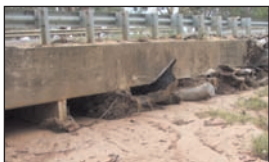
Blocking of flow under bridge
