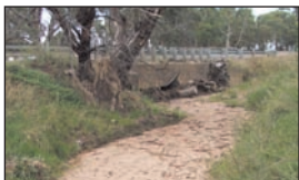
Reducing capacity of drainage
