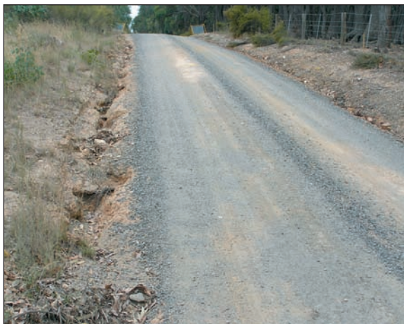
Fig. 14: Gully erosion forming along a road side.
