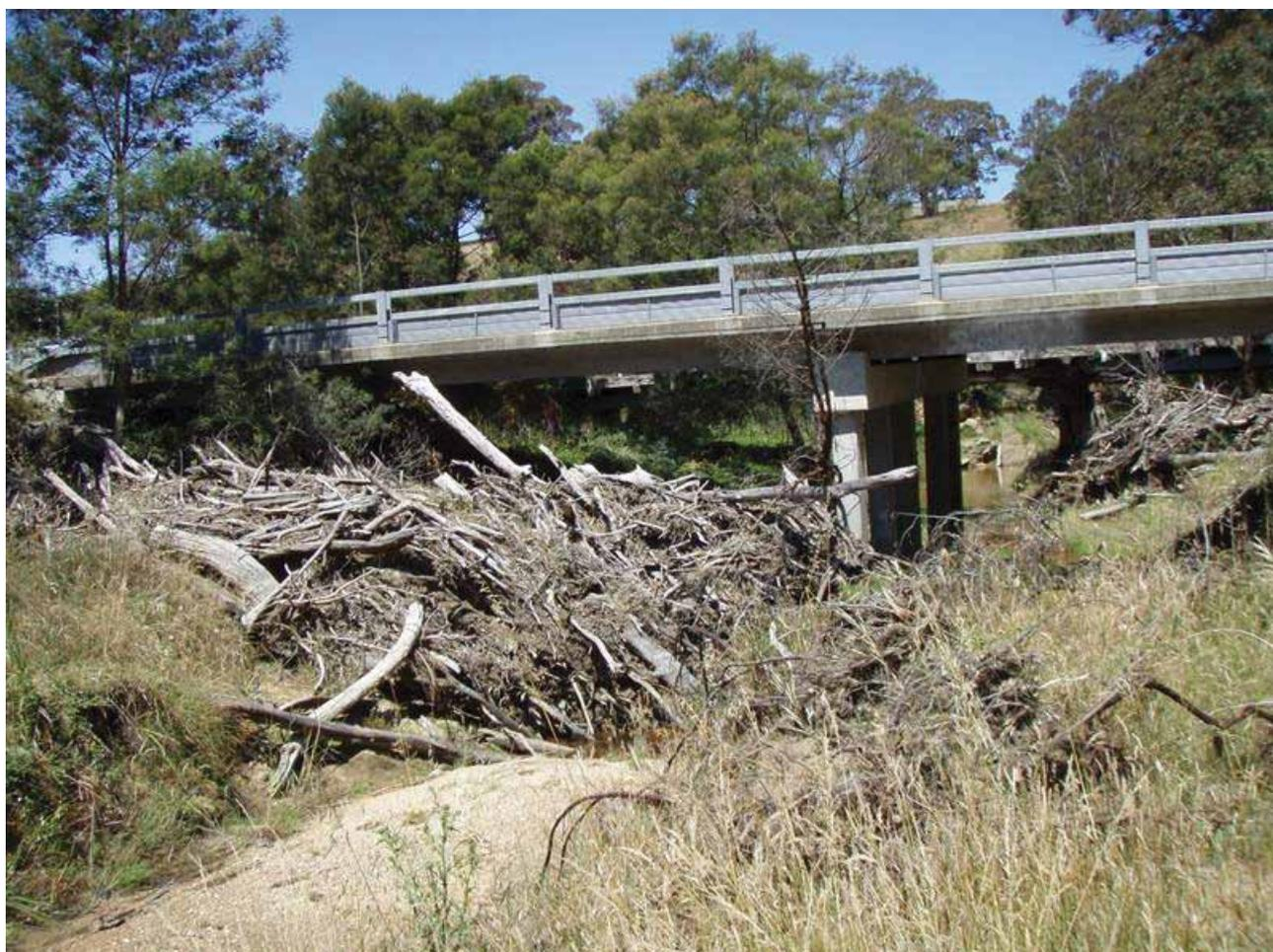
**Figure 7. Large wood trapped against a bridge on Sutherland Creek.** Source: Corangamite CMA
