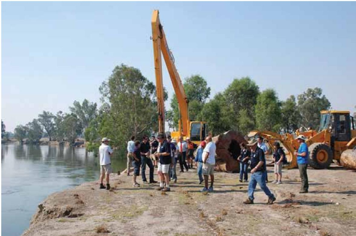
**Figure 6: Resnagging on the Murray River, with large hollow logs being returned for fish habitat and flow diversity.** *Source: Fern Hames*
