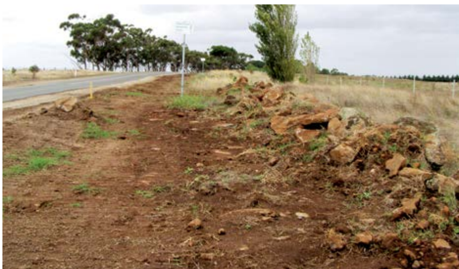
ABOVE: Roadworks impacting on a significant roadside
